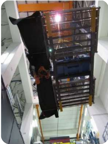
Hoisting the equipment on the casing
